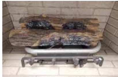
Figure R - Install Middle Log
