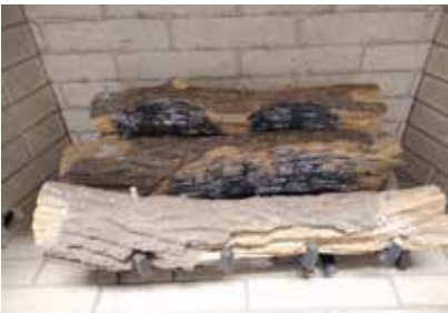
Figure T - Install Front Log
